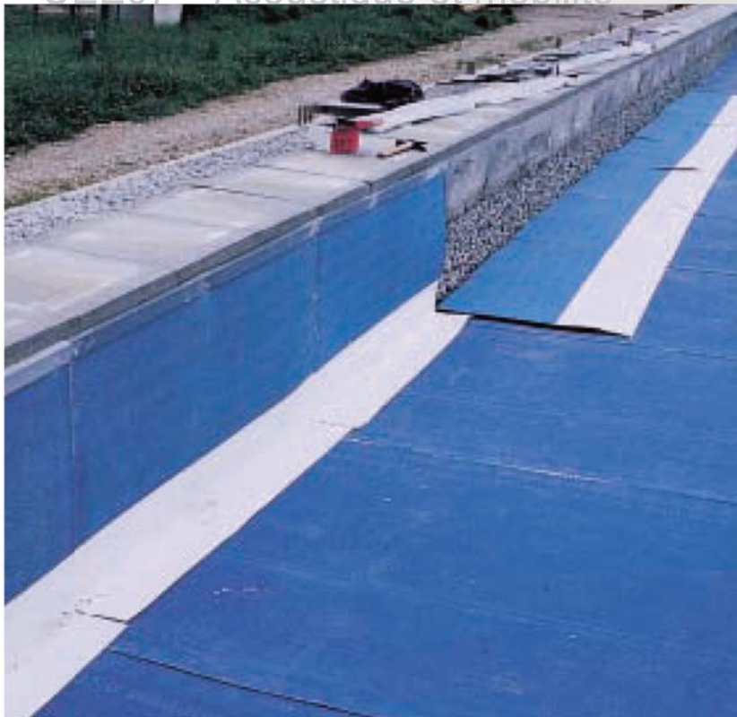
Installation of lateral mats (with special drainage)
